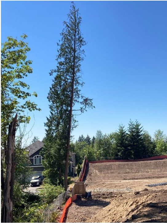
Tree No. 1, showing lean
